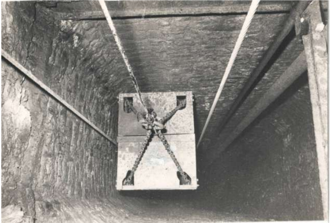
Looking down the main shaft as the cage is lowered. 1977, courtesy of H. Parker
