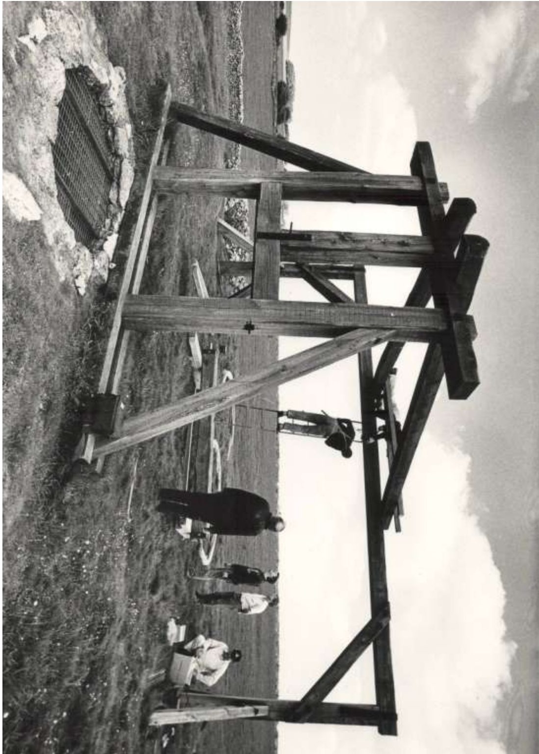
Reconstructing the horse gin, 1988, courtesy of H. Parker
